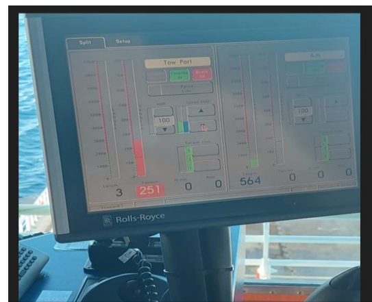
Figure 7. Load Monitor on Vessel
